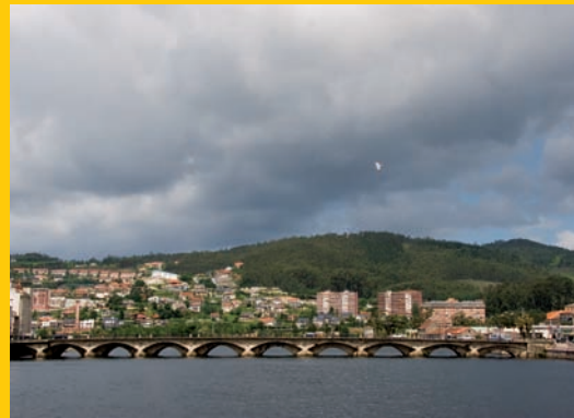
Bridge of O Burgo
